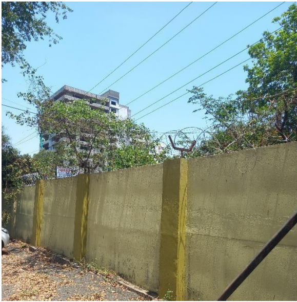
Fencing for Security
