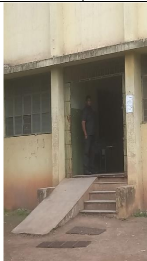
College building ramp
