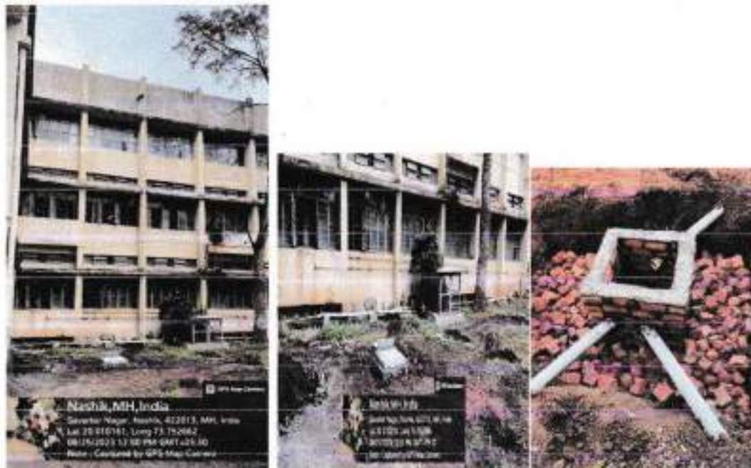
Rain water Harvesting system and recharge pit
