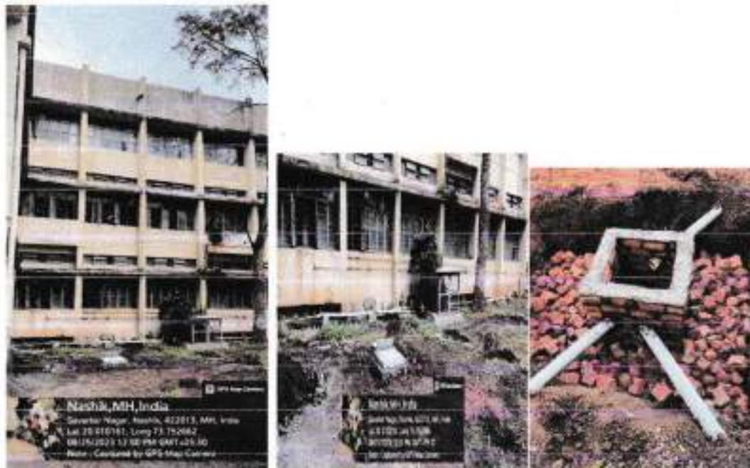
Rain water Harvesting system and recharge pit
